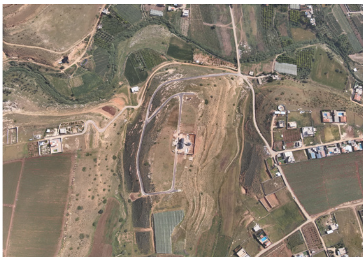
Figure 6: The new road and the beginning of constructions of villas at el-'Unuq (based on an image from govmap.gov.il , accessed on December 2023)
